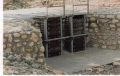
Right: Eastern Lagoon outlet at Banrock Swamp. One of the flow control structures designed by Peter as part of his work for WCA.
